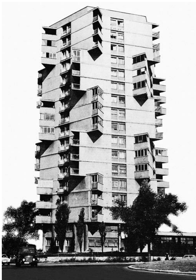
Figure 4. Rista Šekerinski, Residential tower for professors of University of Belgrade in Mitropolita Petra Street, Belgrade, Serbia, 1966. (author's private collection)
