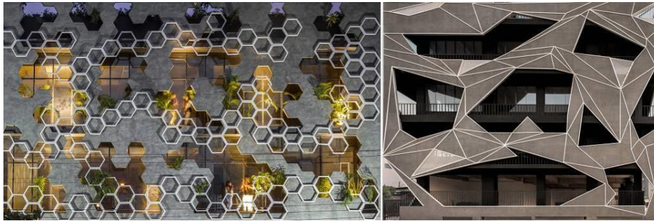
Fig. 5 Formalistic approach to the application of the concept of surface depth: Hexalace, Mohali (Studio Ardete, 2018) (left), Tessalace Commercial Office Space, Mohali (Studio Ardete, 2021) (right) (Source: www.archdaily.com )
